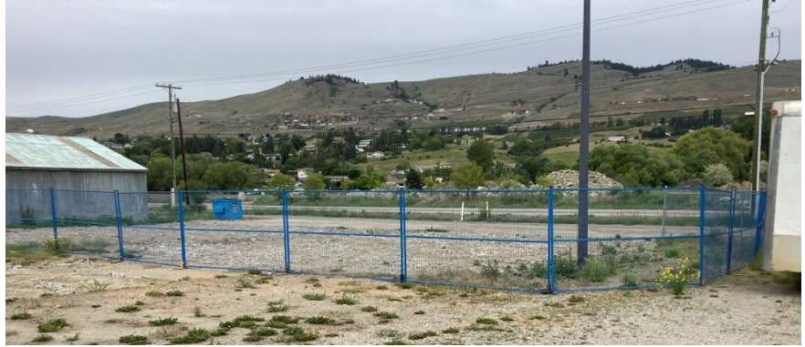
Campbell's are building a hangar off the North Taxiway
